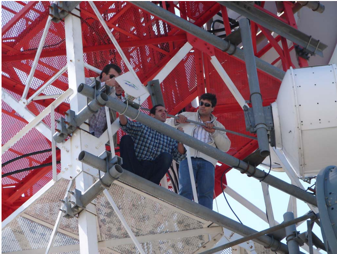
Fig. 8: BreezeNET B equipment at the repeater station (in the Gardunha back-to-back relay).
