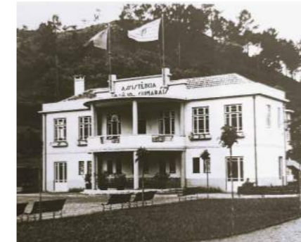
Photo of the building Assistência Araújo Guimarães when it was in operation
