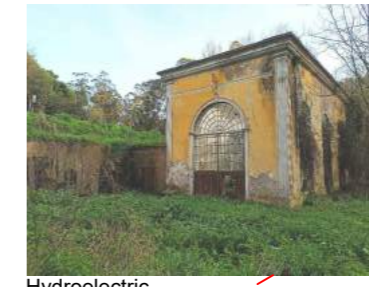
Hydroelectric Power Station
