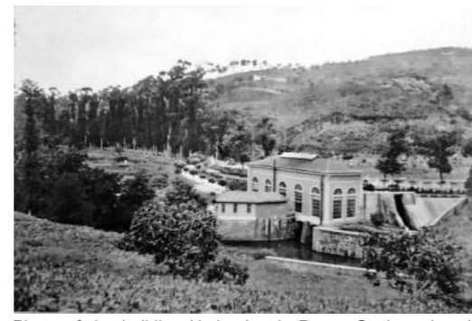
Photo of the building Hydroelectric Power Station when it was in operation
