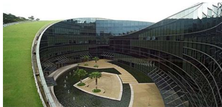
Imagem 20 | Green Roof Art School in Singapore [29] © Perkins+Will/Open Architecture Network
