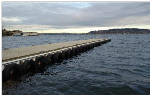
Figure 36 - Dock with Tire Fender System [70].
