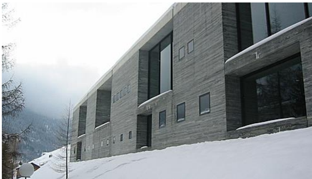
Fig.9 - Fachada exterior, Termas Vals.
