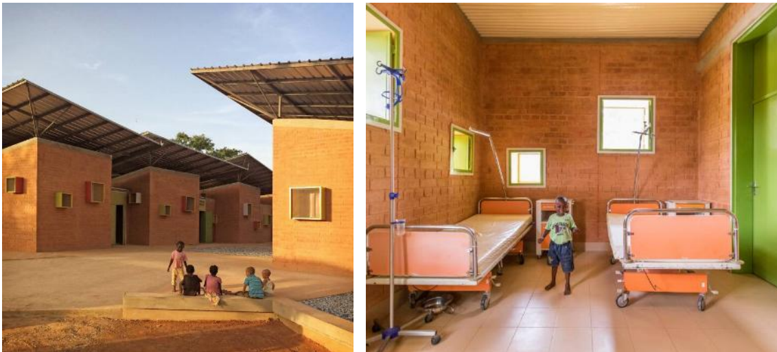
Fig. 16: Léo Surgical Clinic and Health Centre. Fotografias de Kéré Architecture (esquerda) e Andrea Maretti (direita). Fonte – [internet] Disponível em: https://www.kerearchitecture.com/work/building/surgical-clinic-and-health-centre
