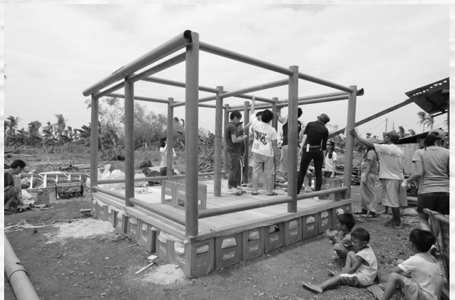
Figure 15 – Volunteers building Paper House Log
