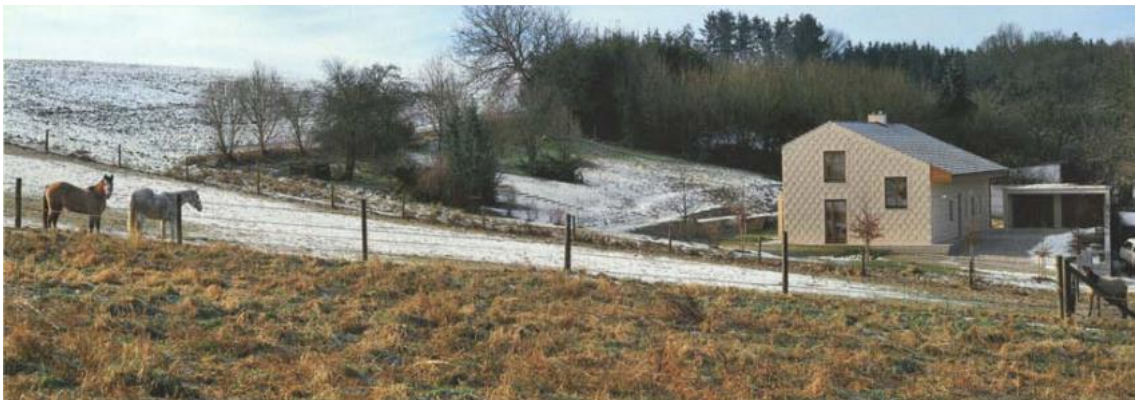
Fig. 43 Private residence (Aggstell, Germany)
