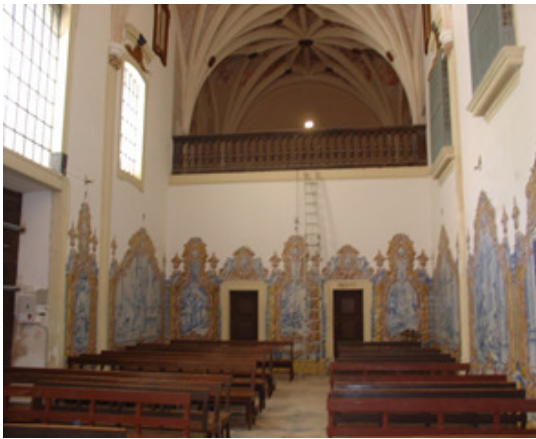
Fig. 5. Higher choir viewed from the nave.
