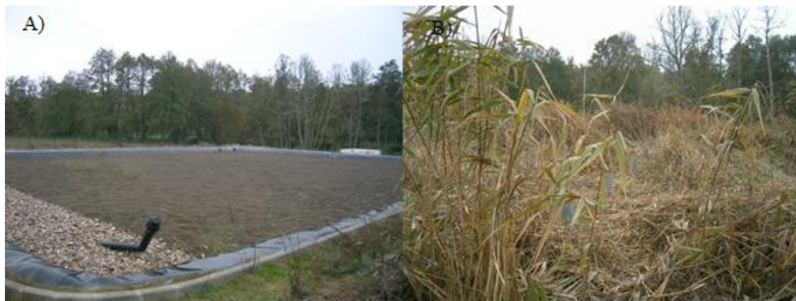
Figure 4.21 - General view of the unvegetated filtration bed of Vila Fernando (A); HSSF-CW bed of Vila Fernando with Phragmites australis (B).
