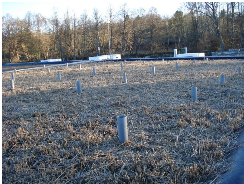
Figure 4.23 - General view of the HSSF-CW bed with measuring points installed.
