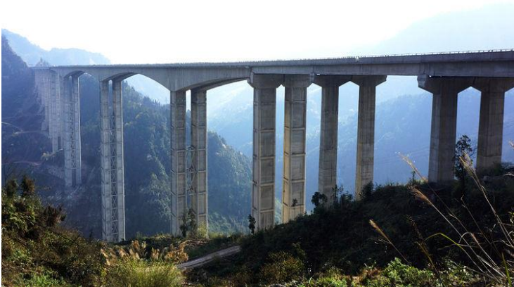
Figure 1.12 Labajin Bridge, pier height of 182.5 m [27]
