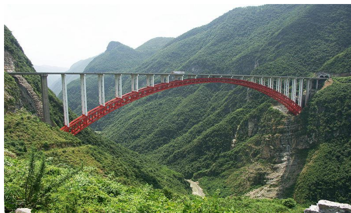
Figure 1.7 Zhijing River Bridge (adapted from [17])
