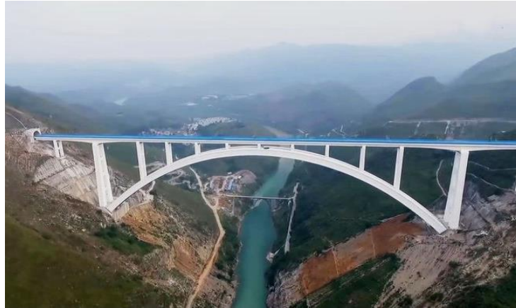
Figure 1.10 Beipanjiang Railway Bridge, with a main span of 445 m [24]
