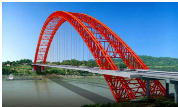
Figure 1.2 The First Hejiang Yangtze River Bridge (adapted from [12])
