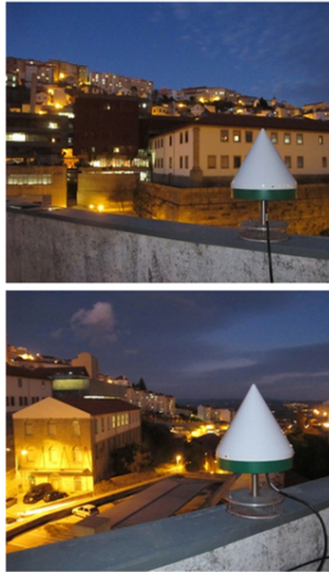
Figure 2.1: Photograph of an antenna from a GNSS station installed at UBI
