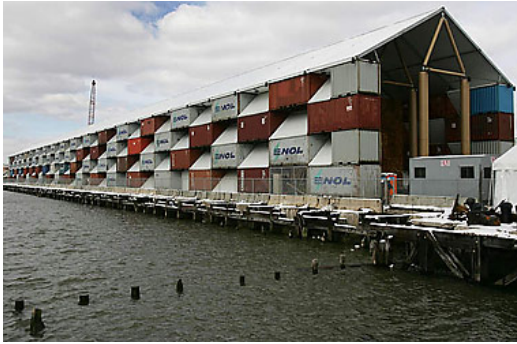
FIG. 33 Exterior do Nomadic Museum de Shigeru Ban Architects (NY, USA) [SBA, 2006] [i14]
