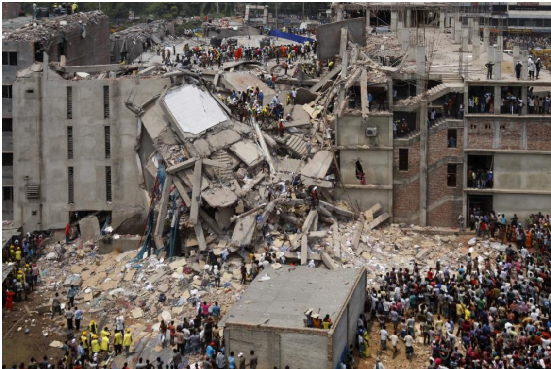
Figure 4. Collapse of the Rana Plaza building in 2013, in Dhaka, Bangladesh (Yardley, 2013).
