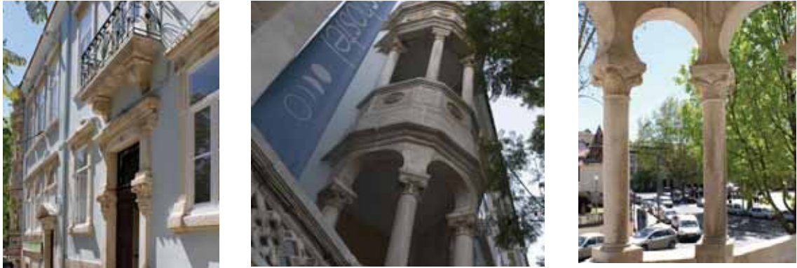
Fig.10 - NS Hostel & Suites, Coimbra
