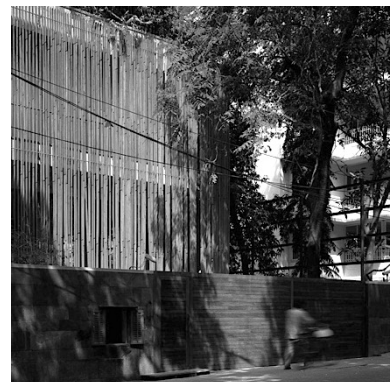
Fig. 4.1.1 - House on Pali Hill, Studio Mumbai
