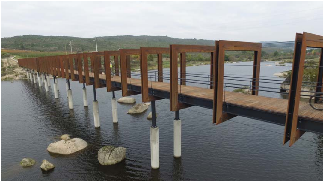
* Ponte pedonal de Ferreirim
