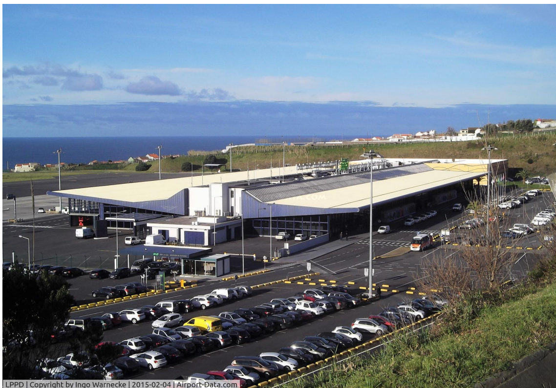
Figure 5.2: João Paulo II Airport, 2015. Photographer: Ingo Warnecke. Source: [81].
