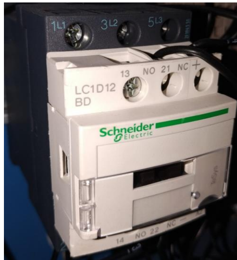
Figura 3.11 - Contactor LC1D12 do fabricante Schneider Electric .
