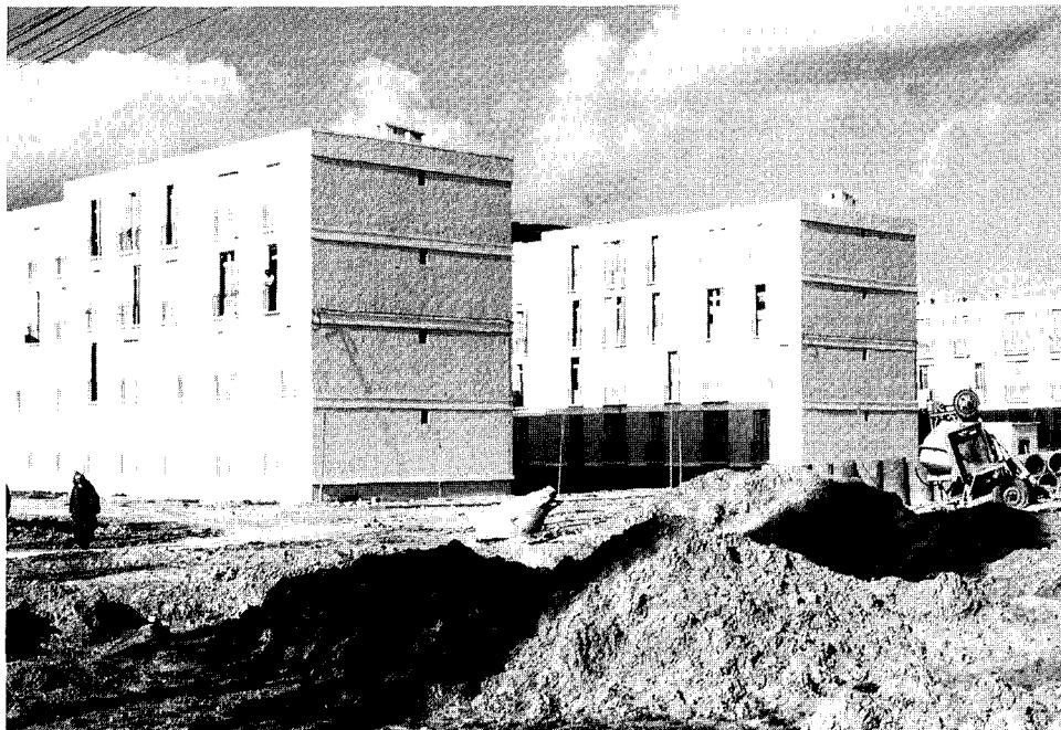
Kasr al-Boukhari, Algeria public housing under construction
