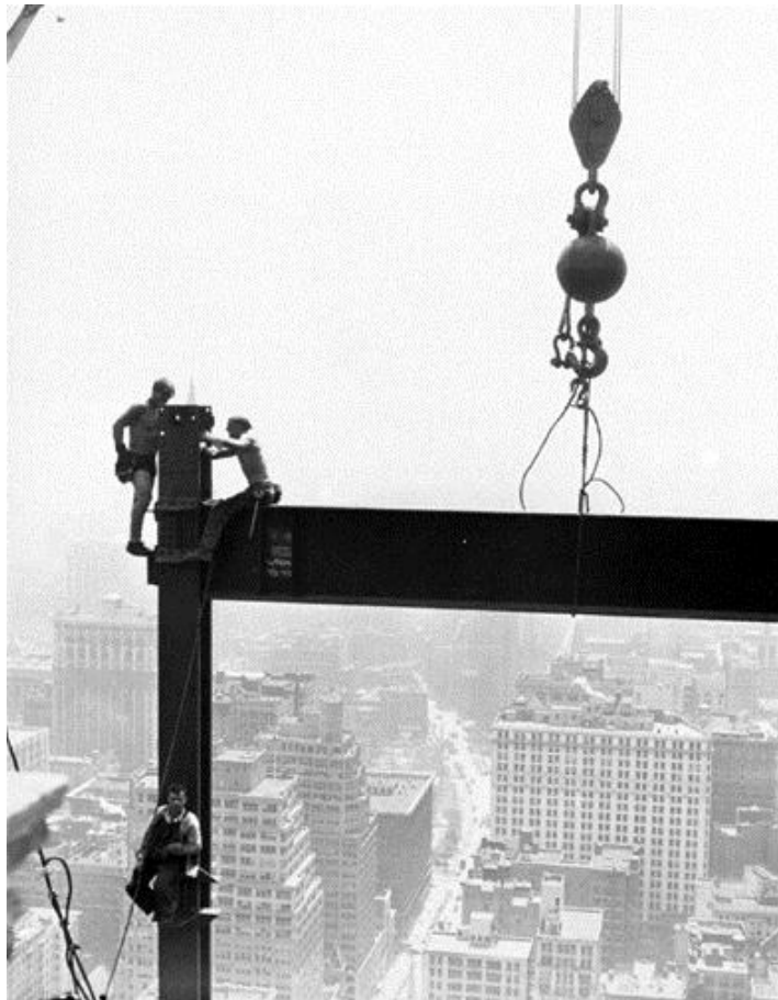
Figura 11 - Laying Beams. Empire State Building Construction, Nova Iorque. 1931. Lewis Hine.
