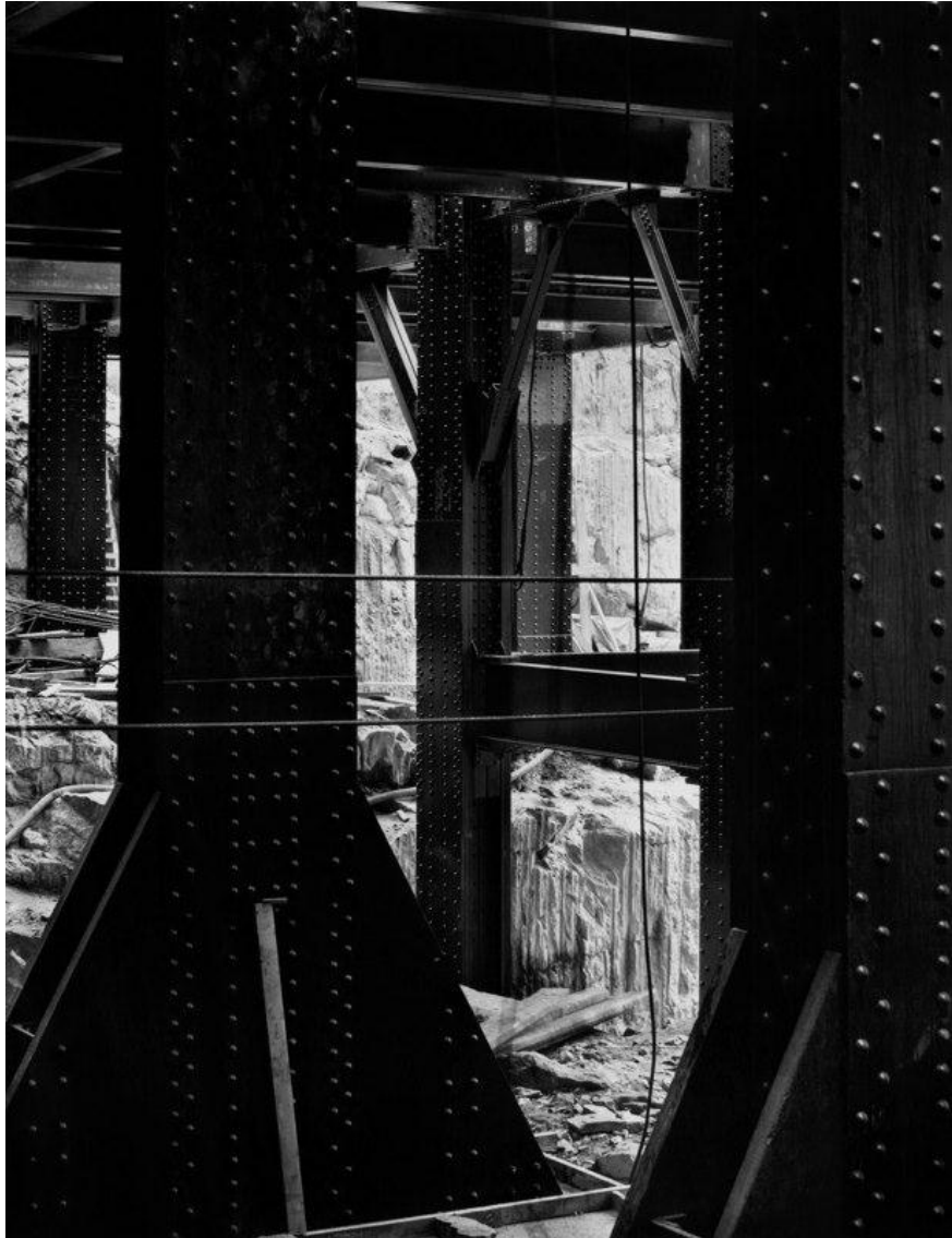
Figura 32 - Foundations of Rockefeller Center. New York. 1932. Berenice Abbott
