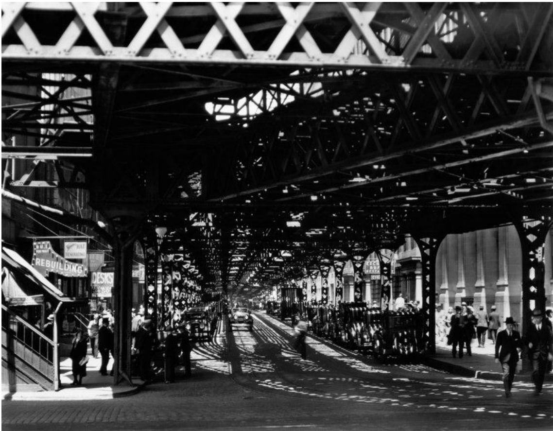
Figura 33 - Under the El at the Battery. New York. 1932. Berenice Abbott
