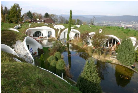
Figura 3.3 - Coberturas ajardinadas - Earth House Estate Lättenstrasse, Dietikon, Switzerland (Architizer, 2013)
