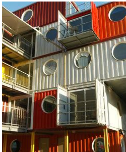
Figura 2.17: Container City II , Londres ([24] Container City).
