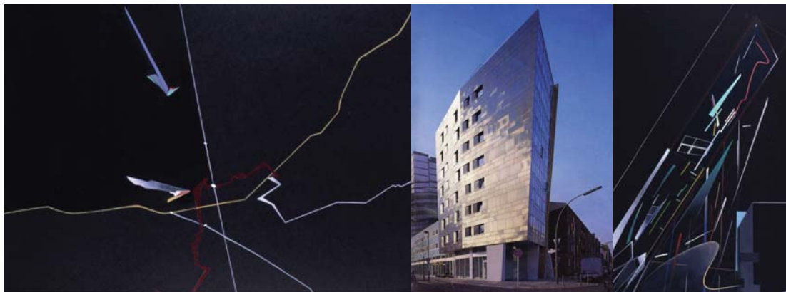
Figura 78 - IBA Housing, Alemanha. Fonte: http://www.zaha-hadid.com/architecture/iba-housing/
