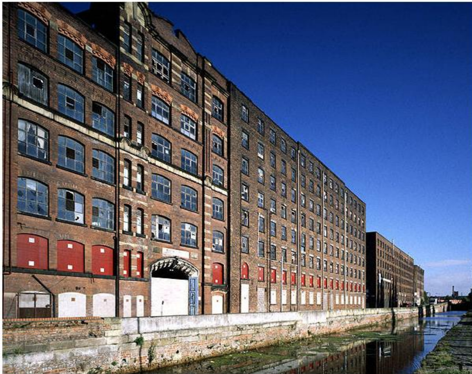
Figura 3 - Manchester, Murrays Mills, Ancoats (Buildings)
