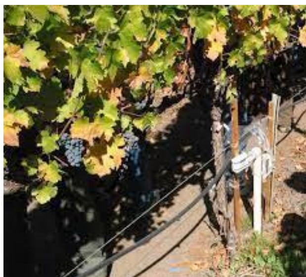
Figure 7. Drip Irrigation system example, when applied to vineyards (Shock, 2013).
