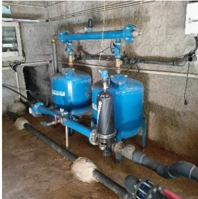
Figure 25. Primary water filtration system before the 1 m 3 water tank, at the Peach Trees field test
