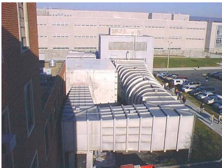
Figura 3.29 - Vista exterior do túnel Virginia Stability Wind Tunnel. (Fonte: http://www.aoe.vt.edu/research/facilities/stabilitytunnel/index.html )
