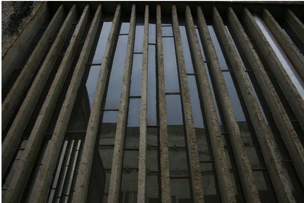
Fig.29 - Vista aproximada dos “Undulating Glass Panes” (www.archdaily.com)
