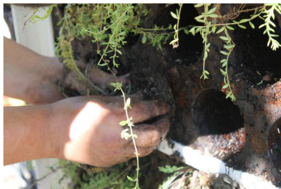
Figure 13 - Plant insertion into the Geogreen module in vertical positioning
