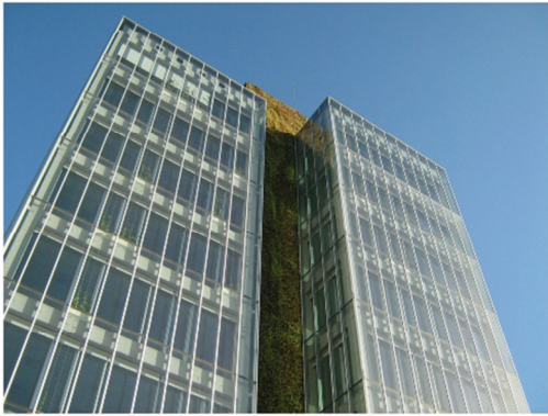
Fig. 5. Modular living wall system, Natura Towers, Lisbon, August 2012.
