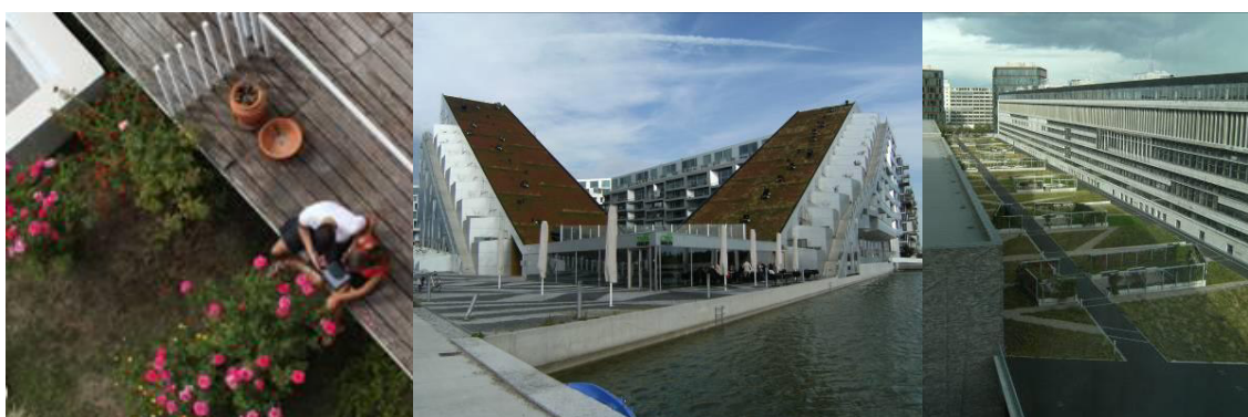
Figure 2 - Private terrace, Torre Verde, Lisboa [39] (left); The 8 Tallen, Copenhagen (September 2012) (middle); Footpath, Copenhagen (September 2012) (right).
