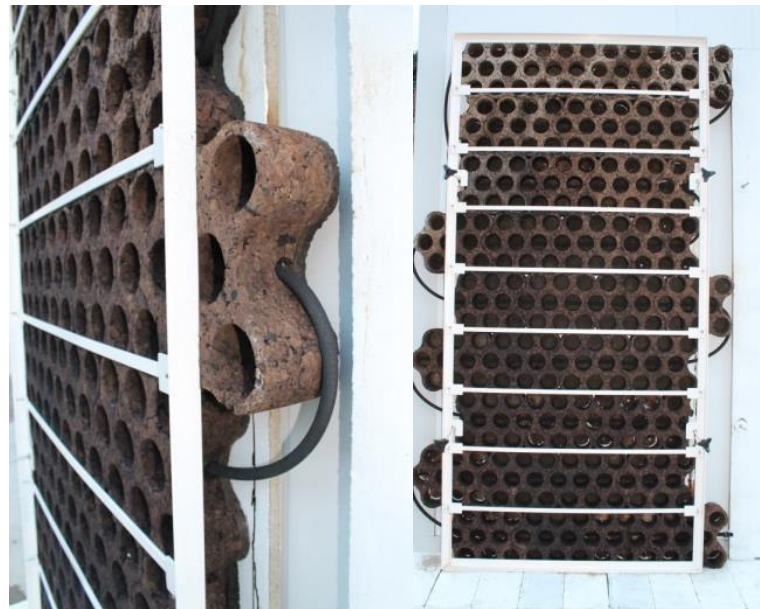
Figure 15 - Geogreen wall irrigation system
