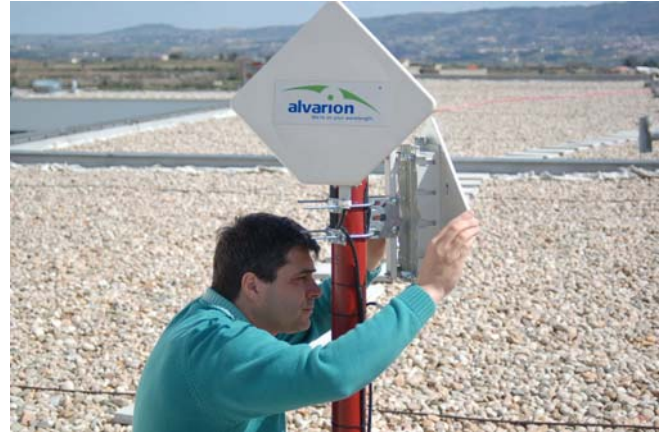
Figure 16: Fine tuning of the antenna tilt.
