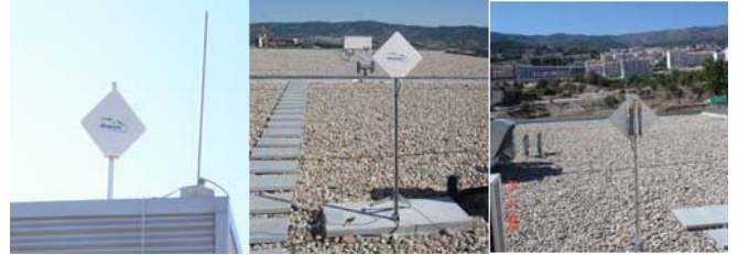
Figure 11: Pilot BreezeNET B installation.
