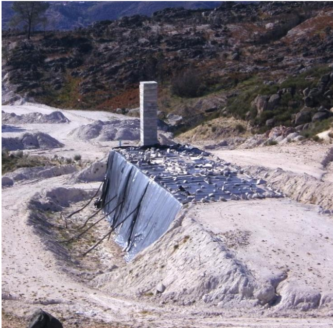
Figure 16. View of the experimental embankment.
