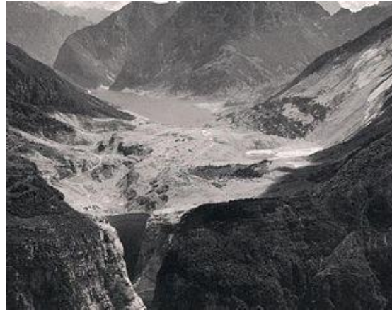
Figure 11. View of the Vajont Dam, Italy, after failure (Petley, 2008).
