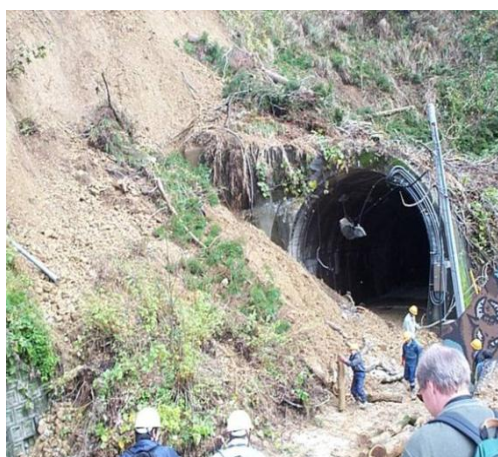
Figure 8. Landslide-blocked west portal of tunnel near the Yamakoshi Village, Japan (Rathje, Jibson et al, 2004).
