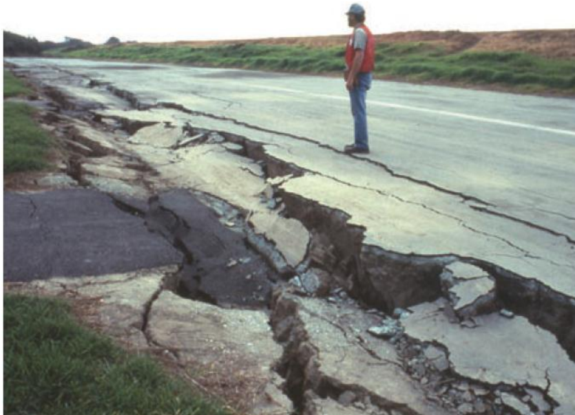
Figure 36. Example of a lateral spread damage to a roadway as a result of an earthquake (Bobrowsky & Highland, 2008).
