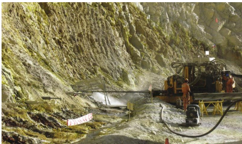
Figure 82. Horizontal drain construction (Read & Stacey, 2009).
