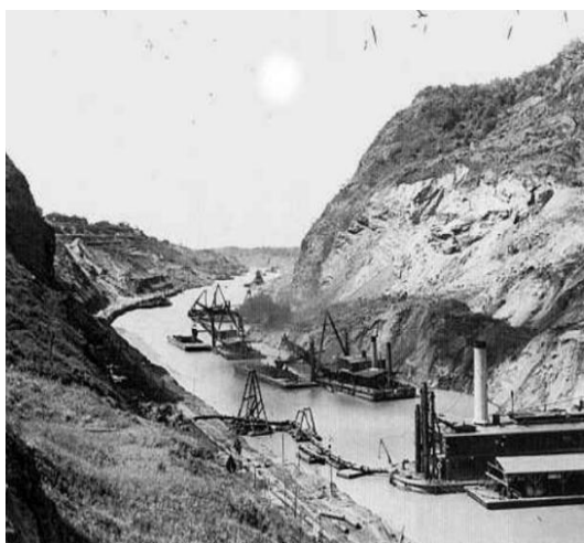
Figure 6. Dredging operations at Culebra Cut 1913 (Rogers, J.; Missouri S&T, 2008).
