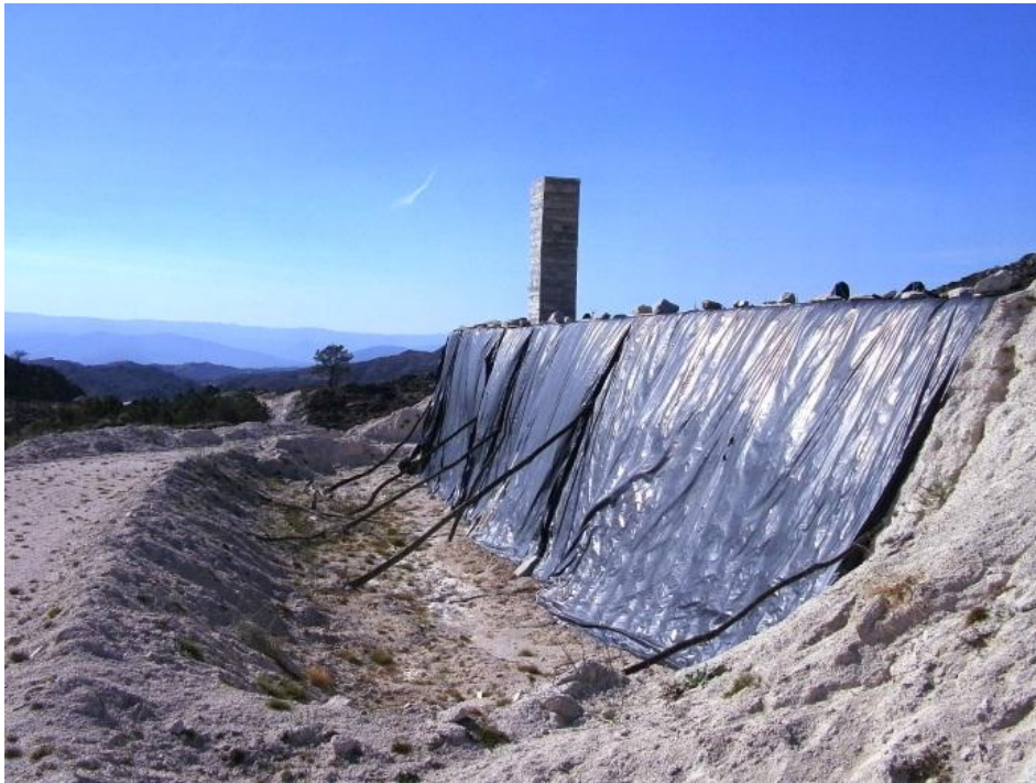
Figure 51. Side view of the embankment shortly after construction.
