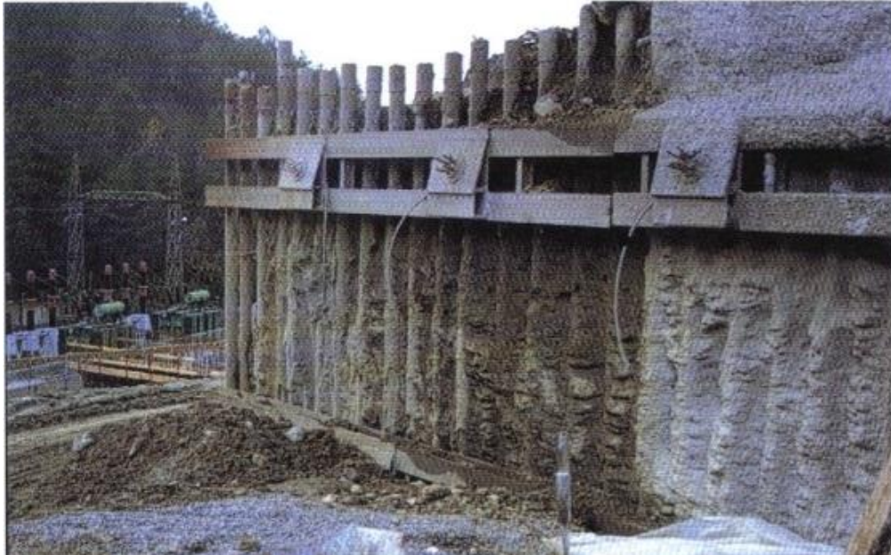
Figure 88. Anchored micropile wall (Vallejo, Ferrer et al., 2004).
