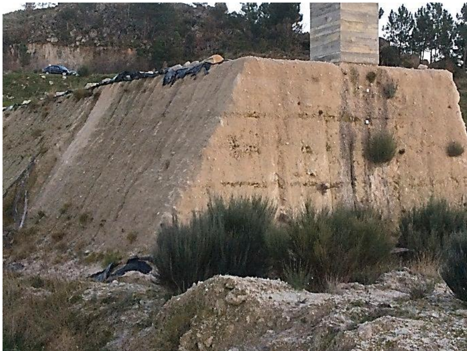
Figure 52. View of the embankment at its current stage.
