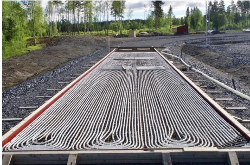
Figure 8: Construction of a solar pavement collector near Östersund, Sweden [75].
