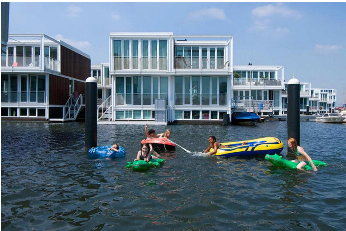
Figura 83| Floating Houses in IJburg, Architectenbureau Marlies Rohmer, Marcel van der Burg (Archaily, 2011)
