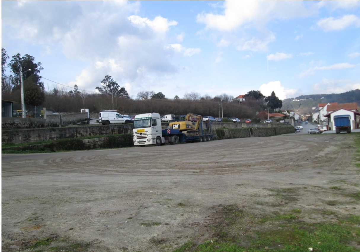
Figure 3. Case study area: two levels of the terrain and the granite retaining wall - Train station surroundings in São Pedro do Sul, Portugal.
