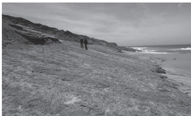
Fig. 2 – Landslide failure in Salgados beach.
