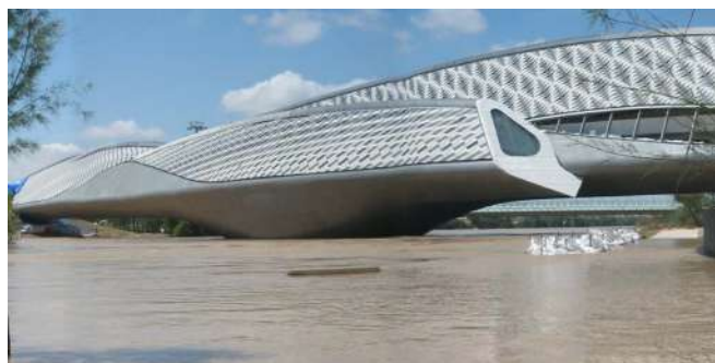
Fig. 1. View from the downstream left bank looking upstream under a flow of 1,500 m 3 /s on June 4, 2008; see the goblet-like covering.
