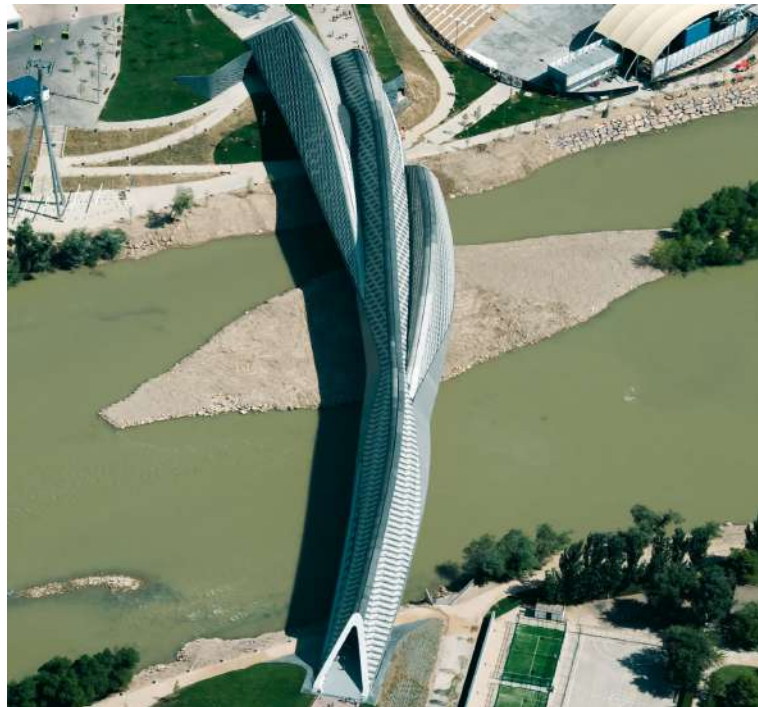
Figure 1.3: Alluvial bar around the bridge, after one of the interventions. [4]
